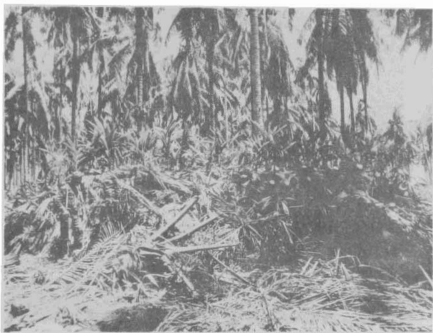
Exterior of typical Japanese bunker. Note soldier on left.
